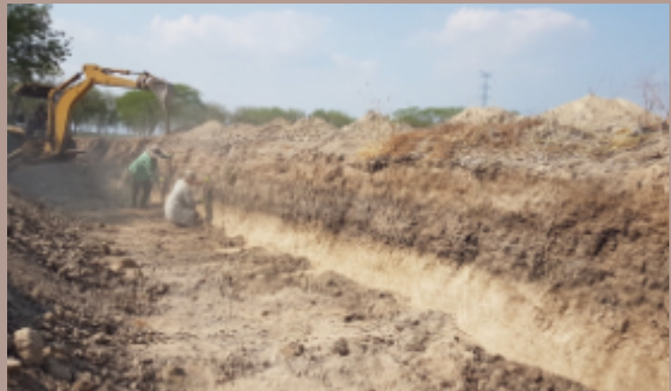
Excavating a paleoseismological trench across the Motagua Fault in Guatemala.
